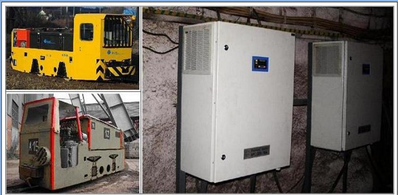
Fig3. Battery charger BPC 144V/130A (Wall mount model, IP-54)
