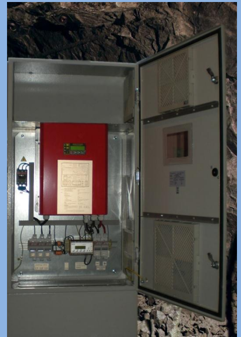
Fig2. The operator panel with LCD display and keypad
